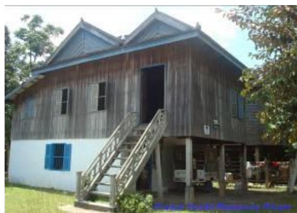
The renovated youth resource room
