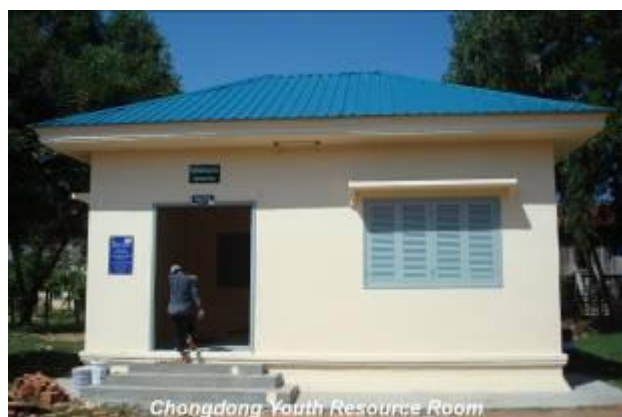
The new build youth resource room
